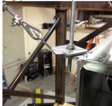
FIGURE 3 – LATERAL SUPPORT COMPONENTS FOR VAV
