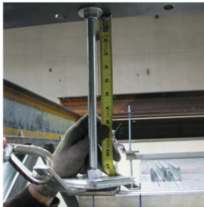
FIGURE 4 – RECOMMENDED LENGTH OF THREADED ROD
